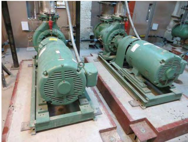
(2) 75 hp pumps, P-2B and P-2B, circulate condenser/boiler water within building 200 (located in #100 penthouse) operate at approximately 30 psi. Pumps are controlled with variable frequency drives. The system can operate with only one motor/pump. These pumps are secondary to the main condenser water pumps listed as separate component.
