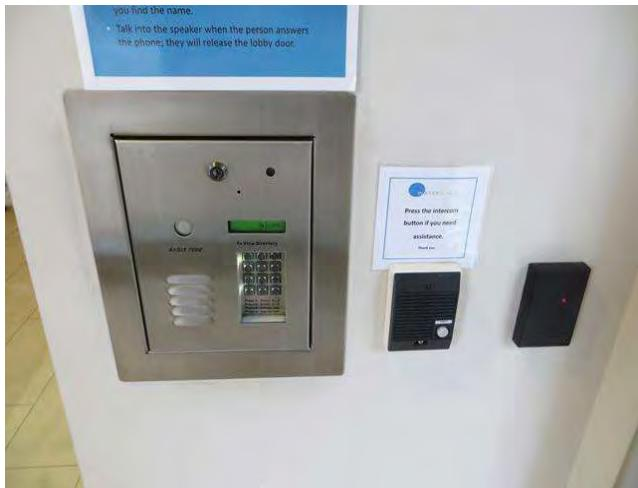
Component covers access control system. Aegis 7000 series allows visitors to call units to gain access to towers.
