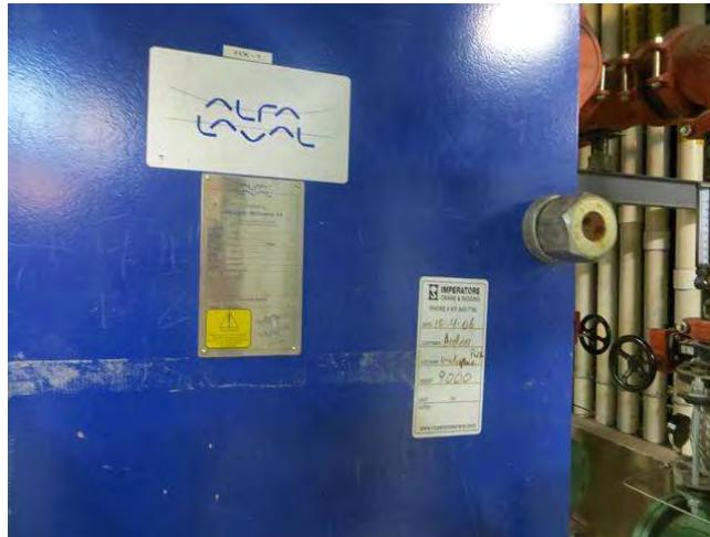
Condenser water heat exchanger provides cooled water to building for air conditioning via water source heat pumps. Cooling tower provides cooled water 75-78 degrees Fahrenheit to heat exchanger. After passing through heat exchanger, condenser water is 80 degrees Fahrenheit maximum.
