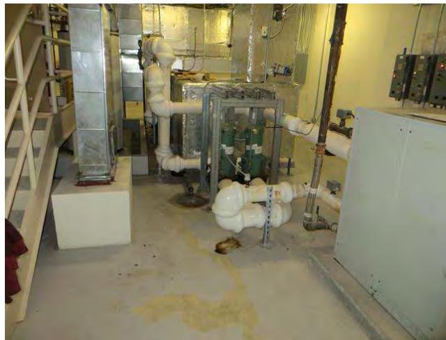
3 hp motor powers Taco 90 GPM circulation pumps servicing McQuay International air handler. Circulate water between water source heat pump and coils inside air handler. Motors operate at fixed speed. (2) pumps for each tower: Pump 9 & 10 tower B.
