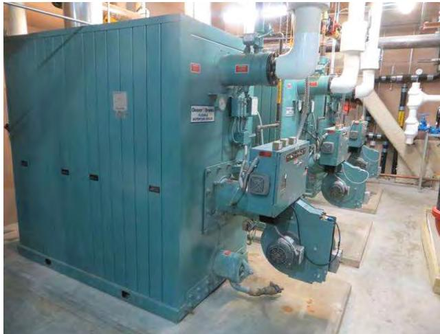
(3) Cleaver Brooks FLX-700-300-160HW gas-fired boilers provide hot water for heating both towers. Capacity is 2400 Mbtu per boiler. Boilers are power-vented through wall to area adjacent to cooling tower.
