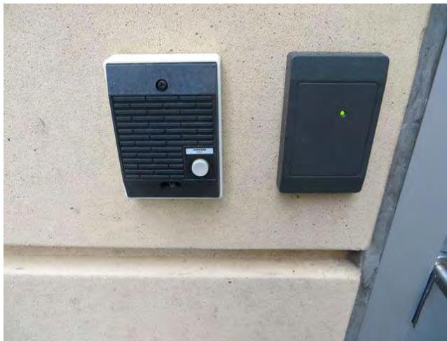
Component covers C.cure 8000 access system. Most components are original. Separate components for intercom system to tower front desks and access dialing system to units.
