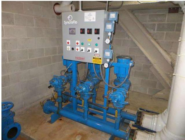
SyncroFlo 55TE74V domestic water triplex booster pumps are powered by 7-1/2 hp motors. 90 gpm per pump.
