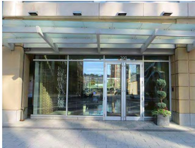
Component covers repair of canopies over tower entry doors. Glass has failed in past due to snow loads. Tower A has two canopies and Tower B has one. Cost provided by client.
