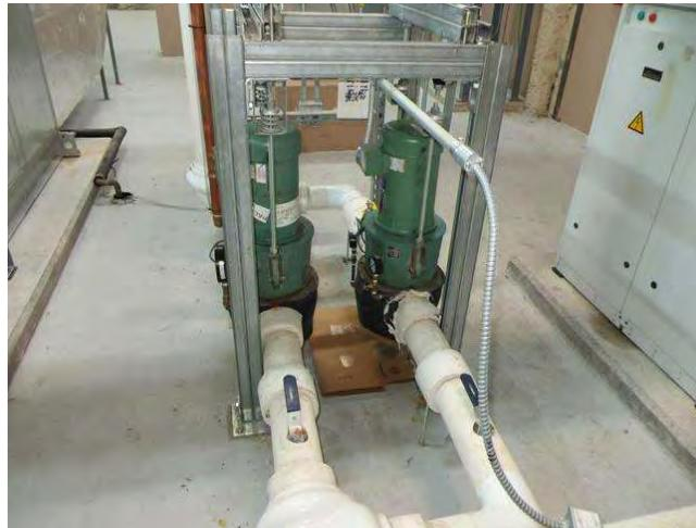
3 hp motor powers Taco 90 GPM circulation pumps servicing McQuay International air handler. Circulate water between water source heat pump and coils inside air handler. Motors operate at fixed speed. (2) pumps for each tower: Pump 7 & 8 tower A
