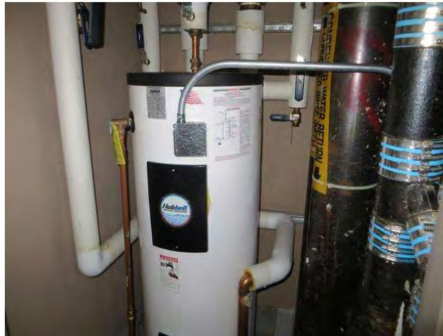
Hubbell 40 gallon electric water heaters have input of 9,000 watts. There is one on second floor of each tower.
