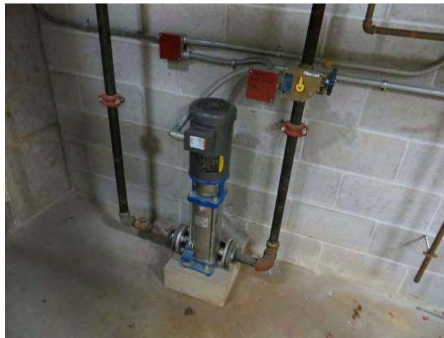
Fire sprinkler jockey pump is in equipment room on level P2 of parking garage.
