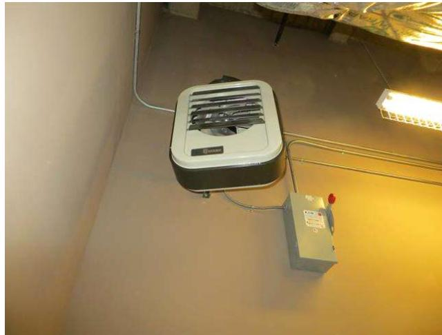
Electrical unit heaters provide heat to mechanical rooms in garage and stair pressurization fan rooms in mechanical penthouses.
