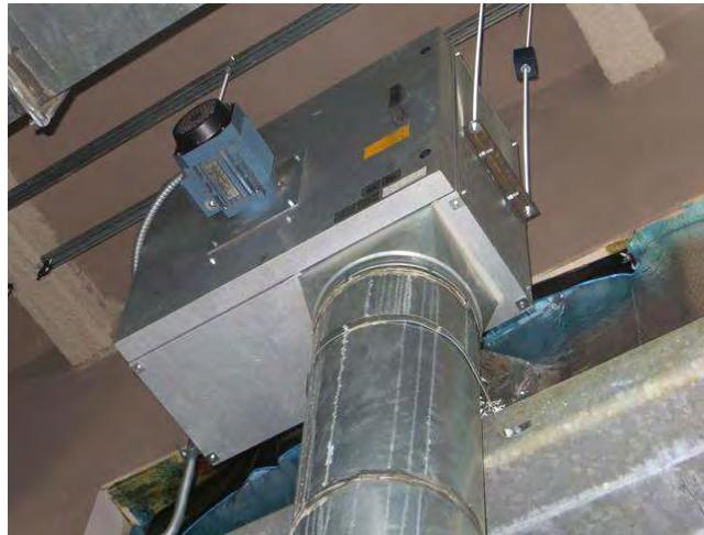
Exhausto fan brings combustion air into penthouse of Tower A for water heaters and boilers.
