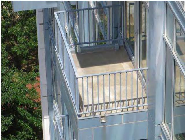
This component covers cleaning and top coating balconies on a 5-year interval. Balcony concrete should be protected from water intrusion to prevent corrosion of reinforcement steel and spalling.
