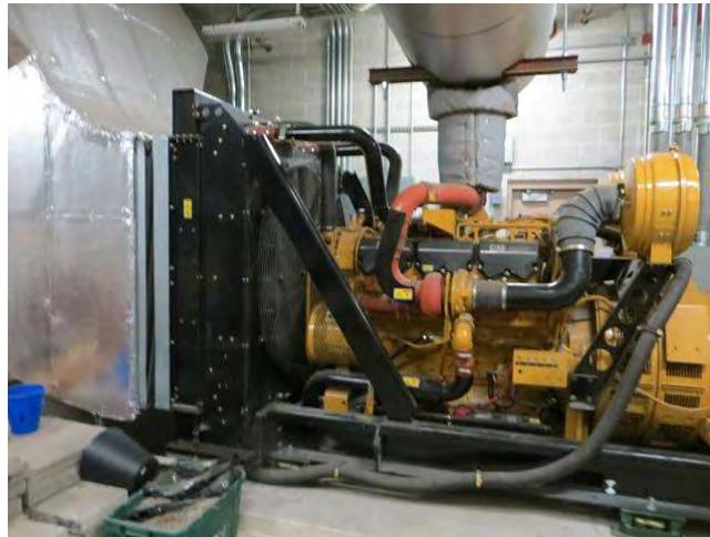
Component covers generator and peripheral equipment. 1000 kw generator has never been needed per client. Waterplace is on same electrical grid as hospital. Power supply has been very reliable. Generator is tested once a week.
