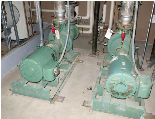
(2) 30 hp pumps, P-1A and P-2A, circulate condenser/boiler water within building 100 operate at approximately 25 psi. Pumps are controlled with variable frequency drives. The system can operate with only one motor/pump. These pumps are secondary to the main condenser water pumps listed as separate component.
