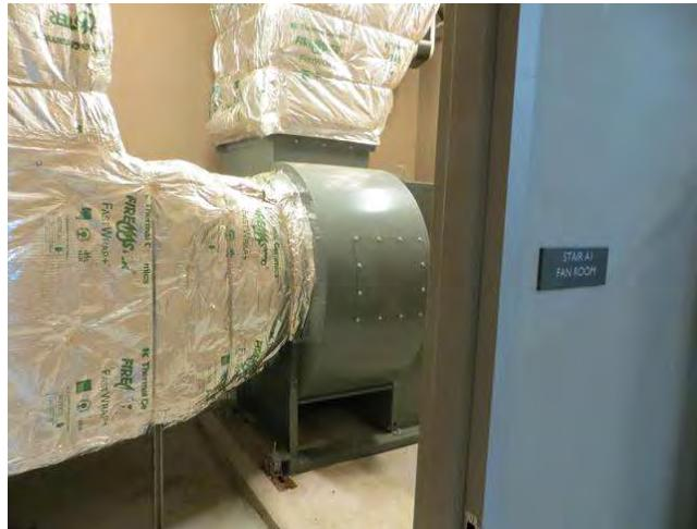
Fire department uses in emergencies to pressurize or depressurize stairwells. Never used operationally.
