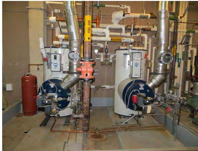
Water is heated to 145 degrees Fahrenheit by PVI main water heaters. Mixing valves in mechanical penthouse temper water to 135 degrees for distribution to building. Hot water is circulated through building to reduce waiting times.
