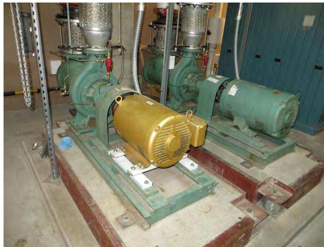
(1) 75 hp pump (P-4) and (1) 50 hp pump (P-3) circulate condenser/boiler water within the boilers and cooling tower. Pumps are controlled with variable frequency drives. The system can operate with only one motor/pump. Secondary building specific water pumps are listed as separate components.
