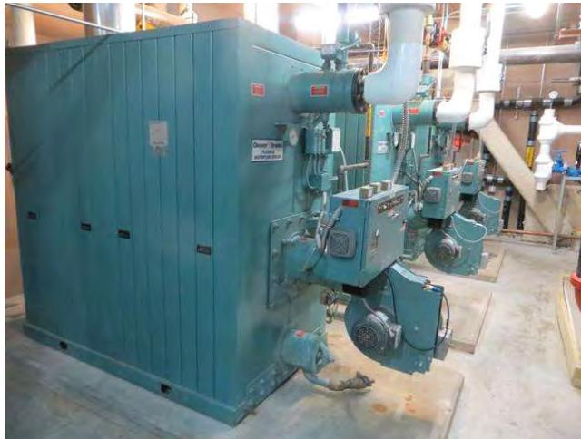
(3) Cleaver Brooks FLX-700-300-160HW gas-fired boilers provide hot water for heating both towers via water-source heat pumps. Component covers scheduled maintenance on 3 year intervals.
