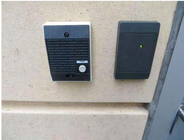
Component covers Aiphone door intercom. Separate components for C.cure access system and access dialing system to units.
