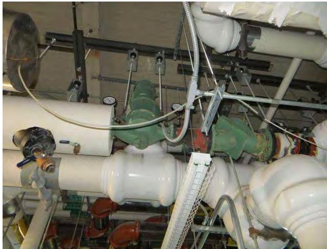
(2) 10 hp pumps (P-11 and P-12) circulate condenser/boiler water within the boilers. Pumps are controlled with variable frequency drives. The system can operate with only one motor/pump. Other condenser water pumps are listed as separate components.
