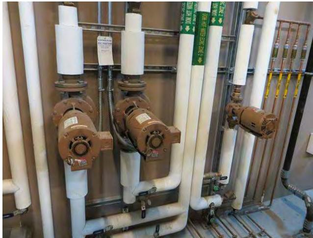
Water is heated to 145 degrees Fahrenheit by PVI main water heaters. Mixing valves in mechanical penthouse temper water to 135 degrees for distribution to building. Hot water is circulated to reduce waiting times. Water for floors 2-10 is pumped both down and up. All of these pumps send water down to building from penthouse.
