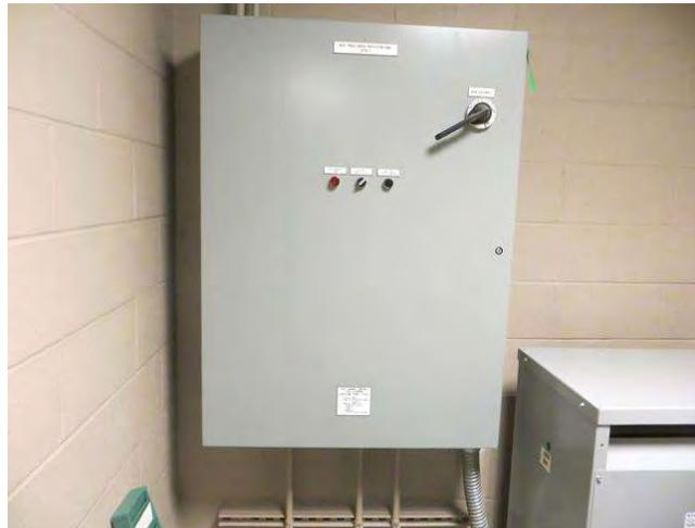
Heat trace system protects elements that contain water from freezing in winter. This includes cooling towers and parking garage piping. There are three control panels in garage and one in Tower A mechanical penthouse. Tyco Thermal Controls is manufacturer.
