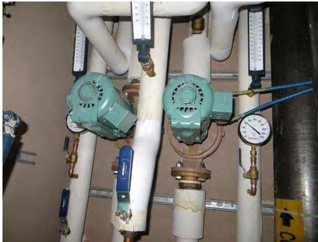
Water is heated to 145 degrees Fahrenheit by PVI main water heaters. Mixing valves in mechanical penthouse temper water to 135 degrees for distribution to building. Hot water is circulated to reduce waiting times. Water for floors 2-10 is pumped both down and up. These pumps send water back up to penthouse. Booster hot water heater on floor 2 is listed as separate component.
