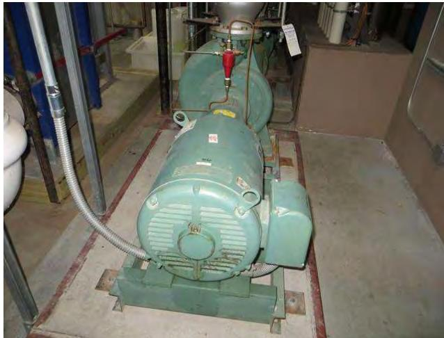
(2) 50 hp pumps circulate condenser/boiler water within the cooling tower and heat exchanger. Pumps are controlled with variable frequency drives. The system can operate with only one motor/pump. Primary and secondary building specific water pumps are listed as separate components.
