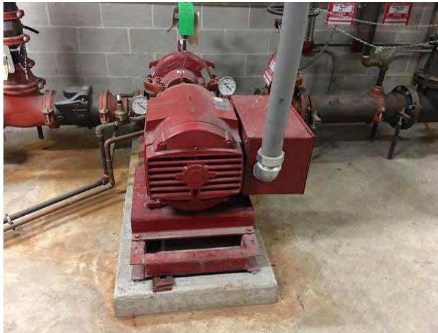
Allis Chalmer fire sprinkler pump is in equipment room on level P2 of parking garage.
