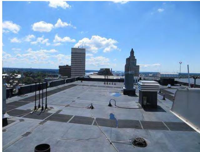
EPDM roof membranes on towers A and B are about halfway through useful life. Roofing quantity calculated from building plans.
