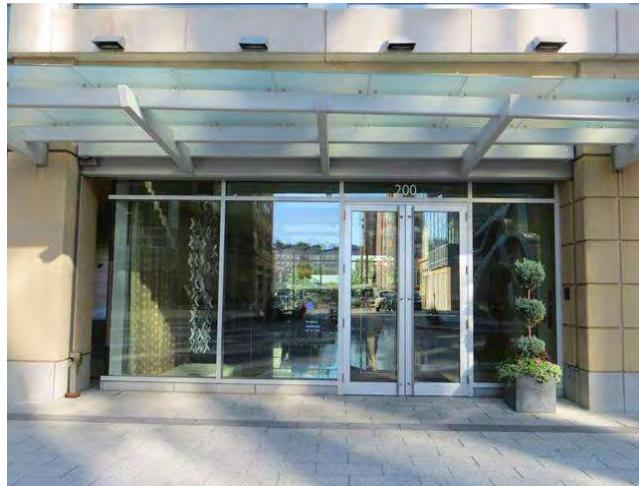
Component represents exterior common storefront window/door areas for both towers on first floor and fitness room on second floor of Tower A. Commercial units on first floor are excluded. Windows and doors were in good condition during site visits and no problems were reported by client.
