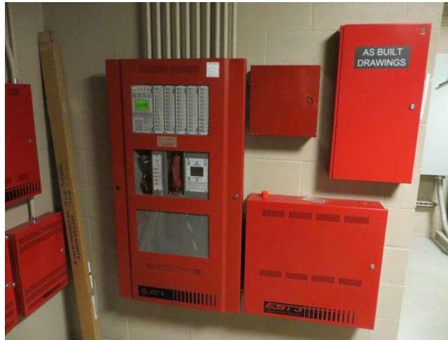
The fire alarm system is composed of Edwards EST3 fire alarm panels and peripheral equipment in the Waterplace towers, garage, and Blue Cross Blue Shield (BCBS) building. Each alarm location has different panel depending on area served. Note that if panels are upgraded in Waterplace and garage, then they also will have to be replaced in BCBS building. Funding for BCBS is not included.
