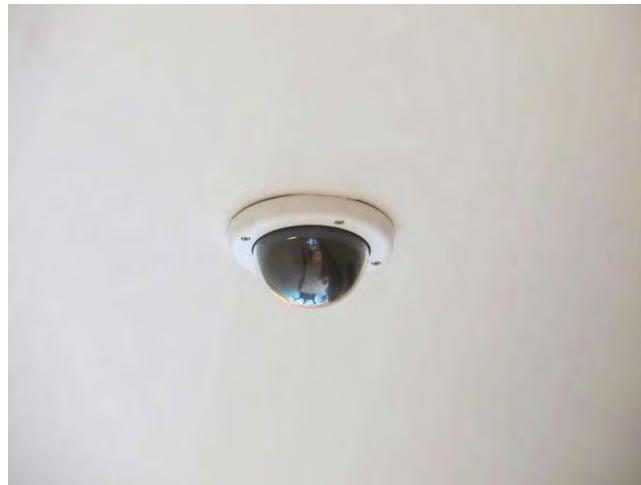
Component covers surveillance system. Original system was analog and lacked detail in camera view. System was upgraded in 2017 with 6 additional cameras and a new DVR/server per client.
