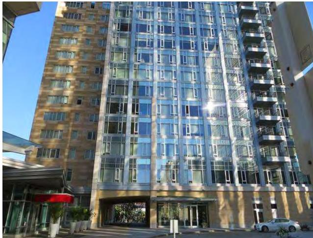
Component represents partial replacement of exterior unit window areas on for both towers. Included are opaque windows and exterior doors on building elevations from floors 2 to the top floor. Cost for this component is 100% association per client. Windows have expected useful life of 30 - 40 years. This component covers replacement of (8) windows at \$7500 every two years at 100% per client. This component should be adjusted as association gains experience with failure rates.
