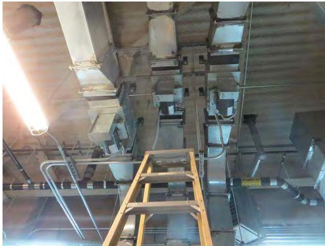
1/2 - 1/6 hp variable speed in line booster fans ventilate unit bathrooms. Quantity from prior reserve study.
